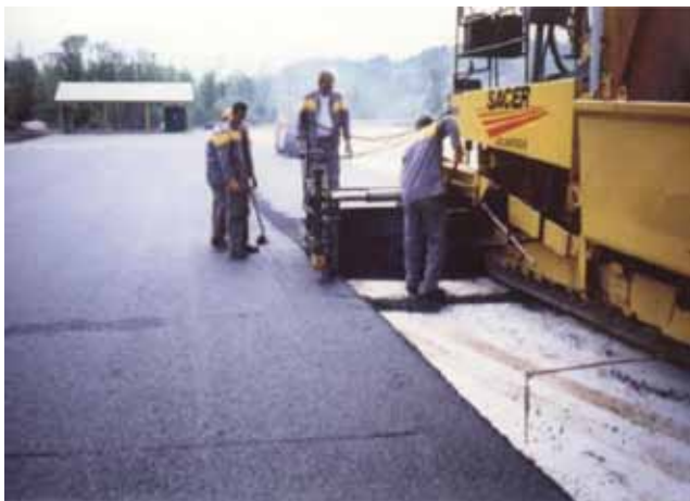
◀ Placement of asphalt on top of COLETANCHE®
