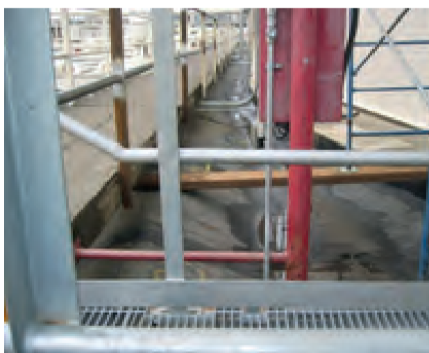
▲ Existing penetrations and obstacles
