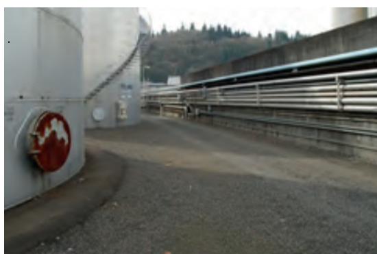
► Terminal before project began
