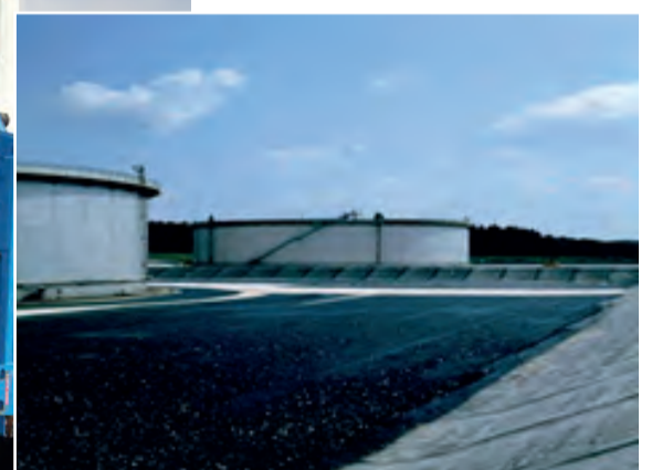
La Mède Total Refinery in France ▲ Asphalt was poured directly on top of Coletanche to provide a driving surface for heavy equipment.
