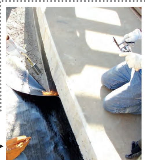
Connecting Coletanche to the concrete ring foundation of the tank ►
