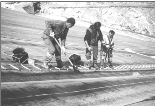
Figure 5. Welding and rolling the joints along the slope
