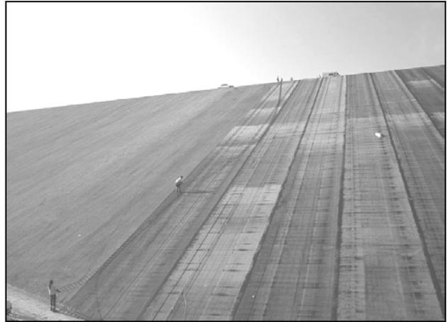
Figure 6. Up to 110-meter long strips of geomembrane to avoid transversal seams
