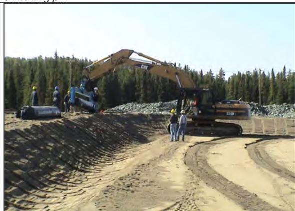
*Distribution of rolls near where they will be installed so that the excavator can pick them up*
