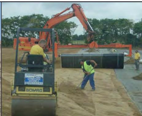
*Excavator with the hydraulic beam offset so the base can be rectified manually just before laying the geomembrane*
