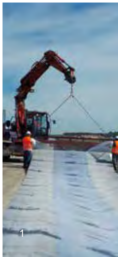
(1) A steel mandrel facilitates unrolling
