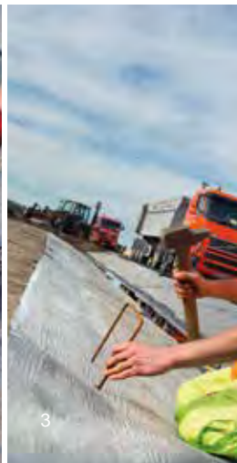
(3) Geomembrane anchored to the ground with a staple
