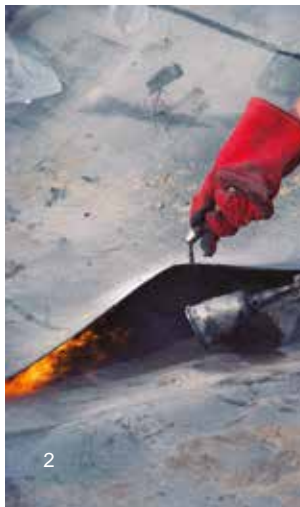
(2) Torch-welded geomembrane
