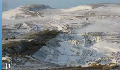
Installation in extreme weather conditions (+40°C)
