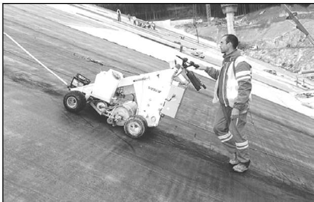
Figure 8. Ultrasonic control by CAC94 equipment
