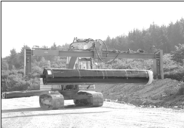
Figure 4. Laying beam and geomembrane roll carried by a 20 tons excavator
