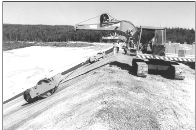
Figure 3. Compaction on the slopes by specially designed equipment
