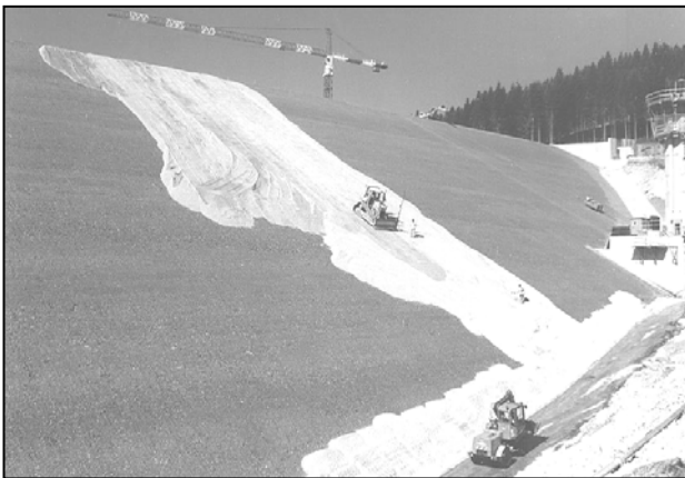
Figure 2. Laying the 0/20 non-bounded gravel as first layer of the waterproofing structure
