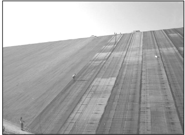
Figure 6. Up to 110-meter long strips of geomembrane to avoid transversal seams
