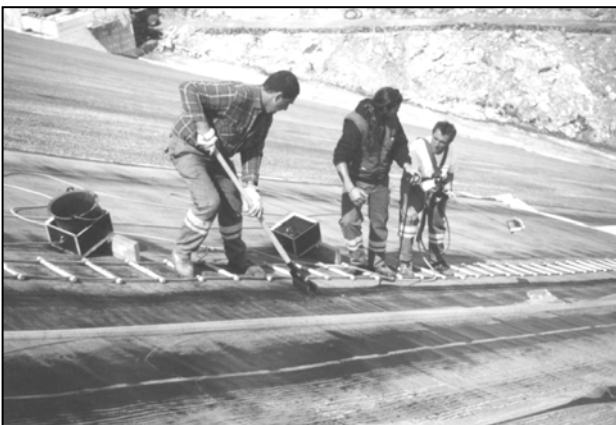
Figure 5. Welding and rolling the joints along the slope
